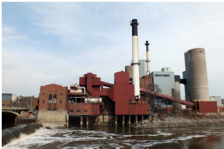
Figure 4.1: The University of Iowa Power plant, located on campus in downtown Iowa City on the Iowa River. From the Little Village article on the University of Iowa's Power Plant [10]
